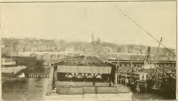
FIG. 6. LOOKING NORTH ON SECTION 3.
